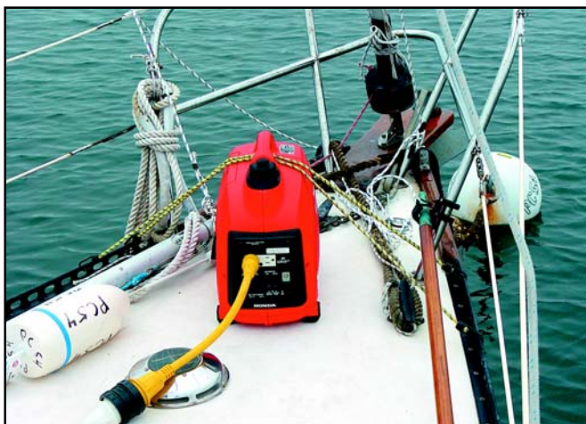
Figure 4—Our little Honda generator keeps the lights on.
